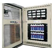
(12 channels, Rack structure )
